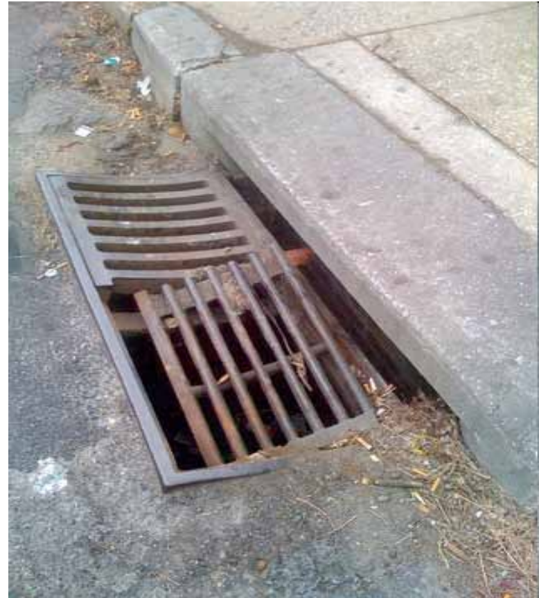
Storm drain system
